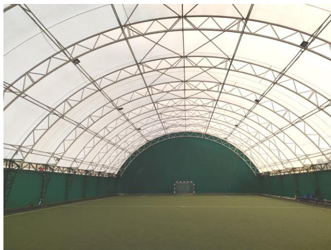
Fig.3. Interior view of the analyzed building in Podgorica
