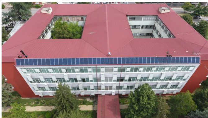
Fig. 4. INNOFEIT Living Lab 30 kW solar power plant
