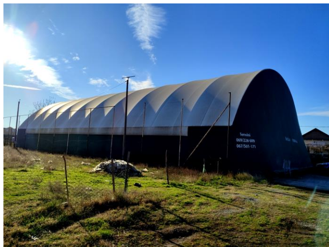
Fig.2. Exterior view of the analyzed building in Podgorica
